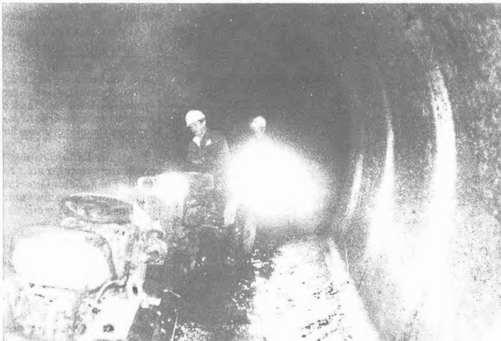
The small tractors used by the contractors inside the tunnel.
